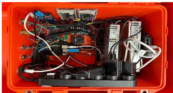
Fig. 3: Low-Level Controller Box
