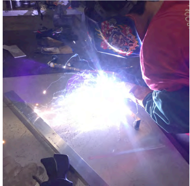
Fig. 4 Nick welding the frame
