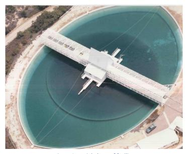
Figure 3: Aerial photo of facility (The bridge structure has no piers or supports in the pond.)
