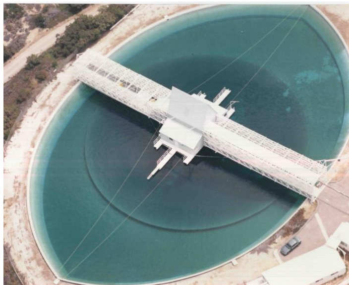
Figure 4: Aerial photo of facility. The bridge structure has no piers or supports in the pond.
