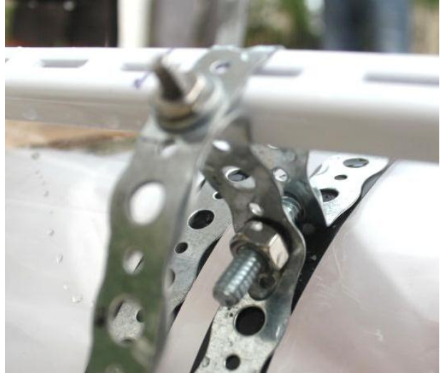
Figure 6. Detail of strap bolting.
