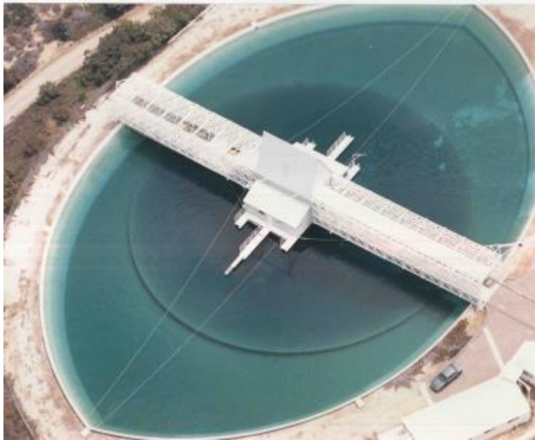
Figure 2: Aerial photo of facility. The bridge structure has no piers or supports in the pond.
