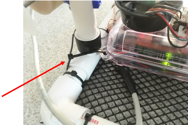
Figure 22 - Photo showing left corner cable ties.
