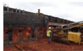
4. Soil Nails—a series of steel bars drilled into the soil, capped at the surface with concrete to create a barrier. $45/sq.ft.
