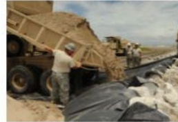
3. Geotextile Membranes – open or closed weave fabric. Natural or synthetic. Coir is woven coconut fibers. Biodegradable and allows for vegetation to grow. $1-5/sq.ft.
