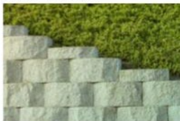
7. Mechanically Stabilized Earth blocks - interlocking blocks set down over reinforced mesh. $15-30/sq.ft.
