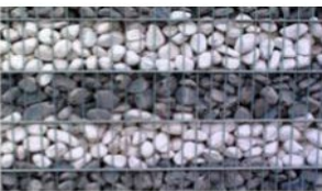
5. Cage System – rocks and boulders in separate wire cages, stacked in place. $5/sq.ft.
