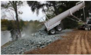
1. Riprap— loose collection of large stones, installed over geotextile membrane. $4-5/sq.ft.
