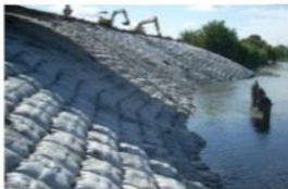
6. Articulated Concrete— form a grid of interconnected units of abutting blocks. $10-20/sq.ft.
