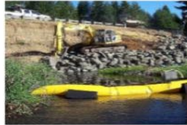
2. Turbidity Barriers – geotextile membranes that float, is anchored with weights. $10/sq.ft.
