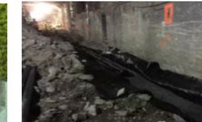
8. French Drain System - underground piping or drain tile that channels water to an exit point. May be perforated. $45/sq.ft.
